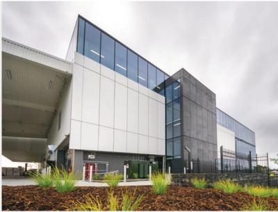
The scope of works included foundations, forming of the building platform and the construction of a three-storey building comprised of pressurised laboratory spaces, controlled pharmaceutical manufacturing areas, write-up spaces, general office and staff facilities, and a canteen on the third level. A new warehouse space connects to the existing facility through a skybridge.
